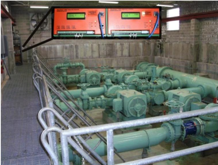
**Photo of the 50MGD Pump Station. Four Sensus Turbo Meters (16 Inch), which were outfitted with ICE® registers, are now monitored by two EtherMeters™. The meters (not shown) are located in a below-grade vault several hundred feet from the pump station. The industrial communication protocol used is MODBUS® TCP.**
